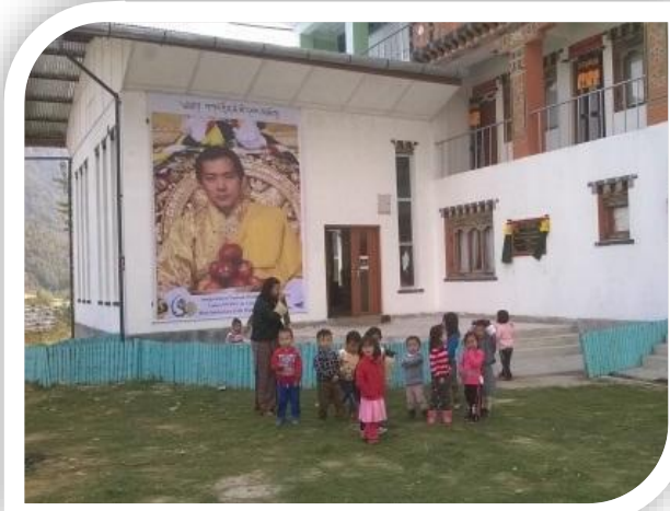
Ground floor: Day-care center
