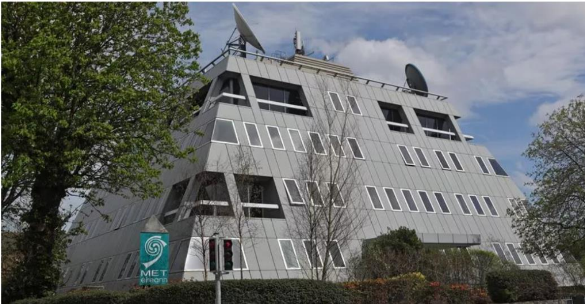
Met Éireann, Headquarters, Glasnevin Dublin, Ireland
