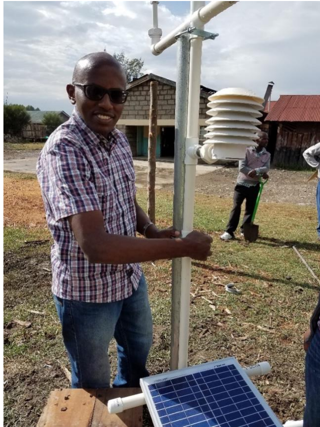
Figure 16.2. Charles Mwangi, Kenyan GLOBE Coordinator, finishing the installation of a 3D-PAWS system located at the Magomano Girls High School, Kenya.
