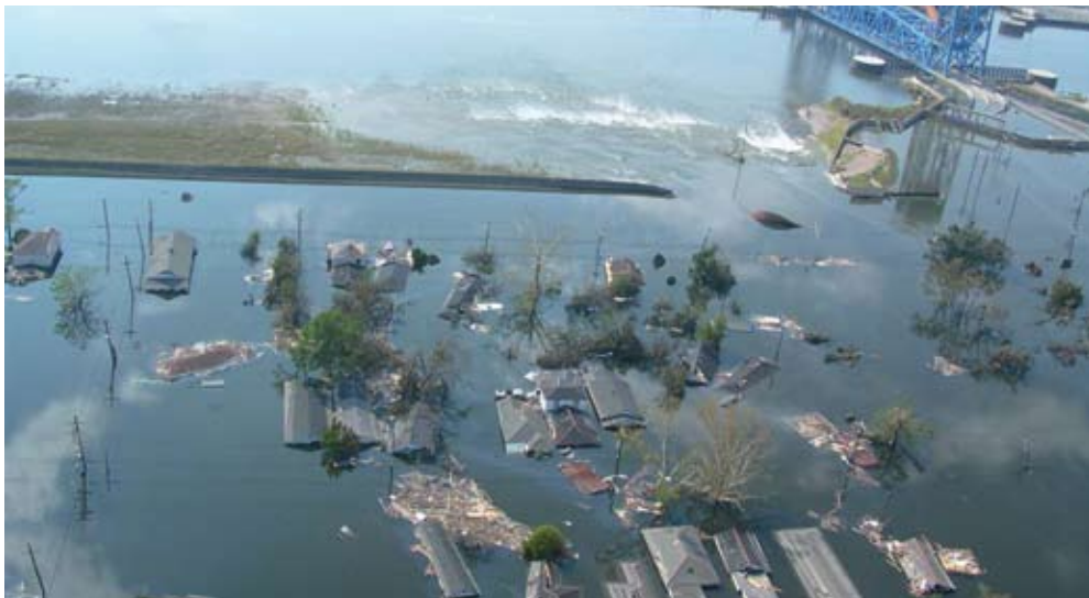
Figure 5.4 Industrial Canal, East Bank, North Breach
