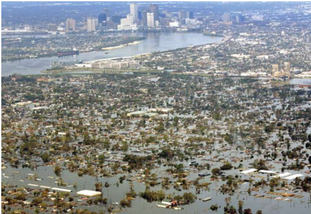
Figure 5.9 New Orleans Flooded
