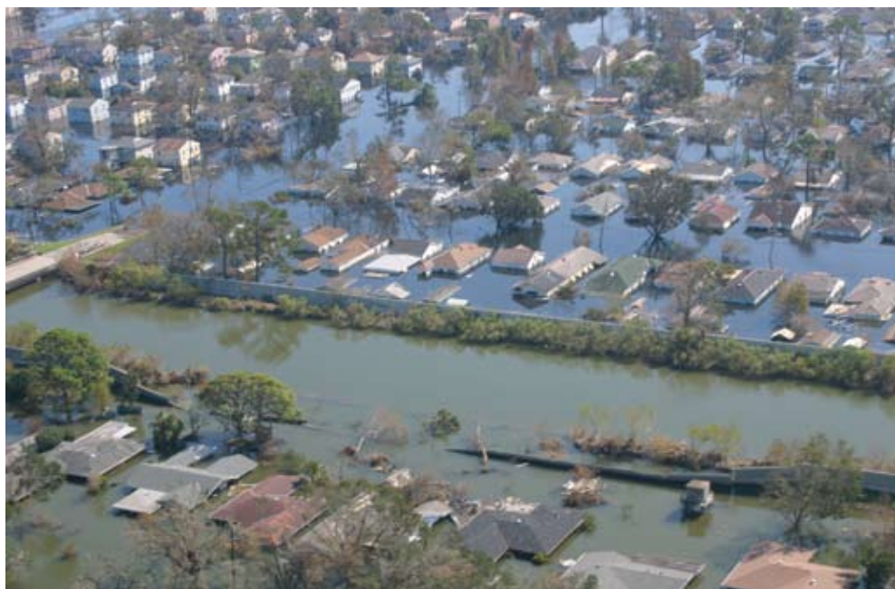
Figure 5.8 London Avenue Canal North Breach
