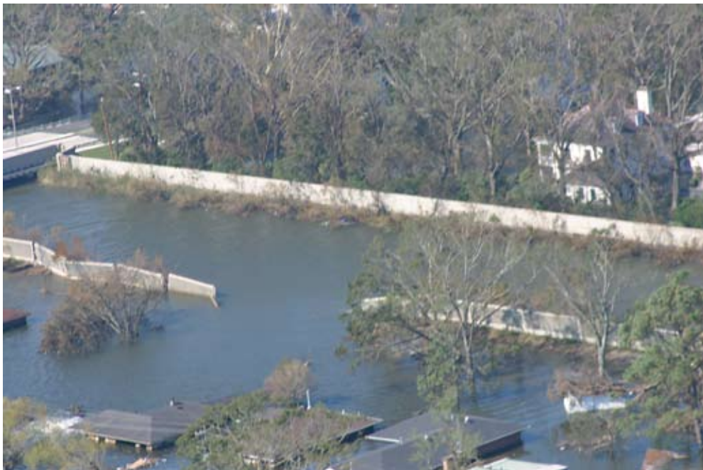
Figure 5.6 London Avenue Canal South Breach
