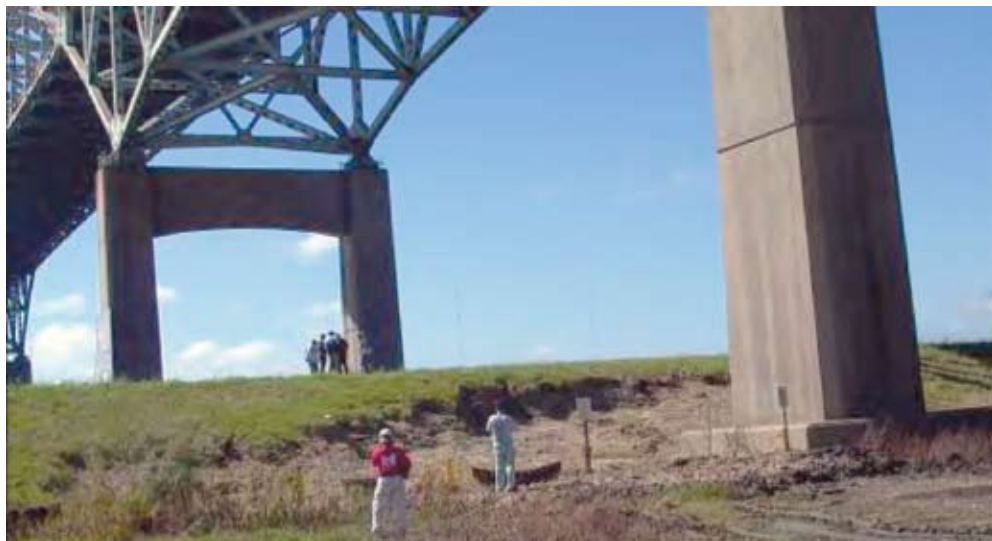
Figure 7.11 Levee Under the Paris Road Bridge in New Orleans East
