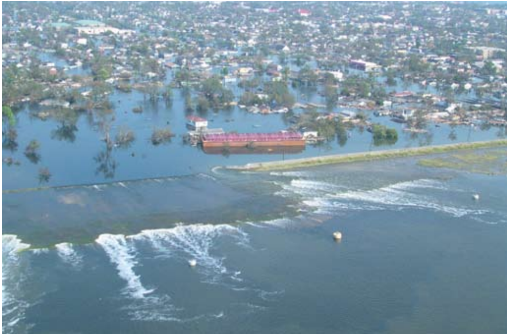
Figure 5.5 Industrial Canal, East Bank, South Breach
