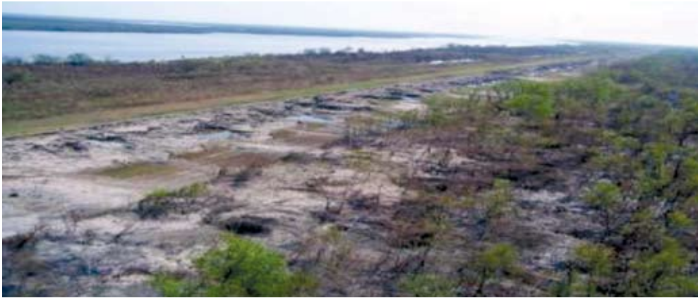
Figure 7.12 Obliterated Levee along the Mississippi River-Gulf Outlet
