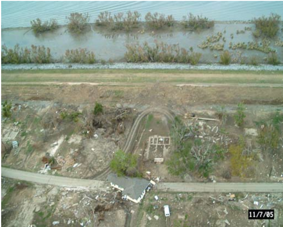
Figure 5.2 Hurricane Damage in Plaquemines Parish
