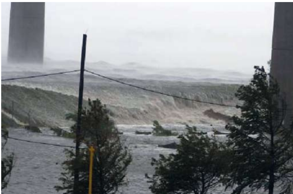
Entergy Corporation personnel took this photo of storm surge waters cascading over a levee near the Entergy power plant in the New Orleans East area.
