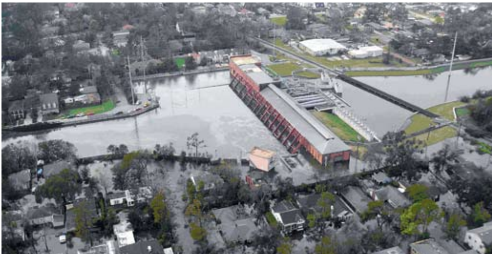
Figure 5.11 Submerged Pump Station No. 6
