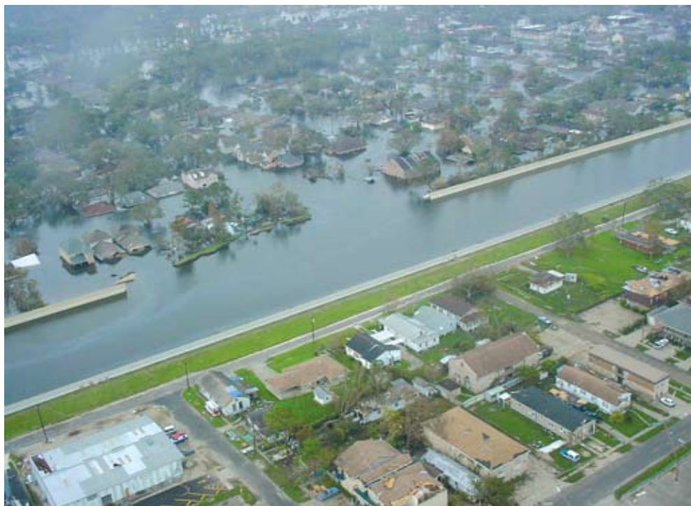
Figure 5.7 17th Street Canal Breach
