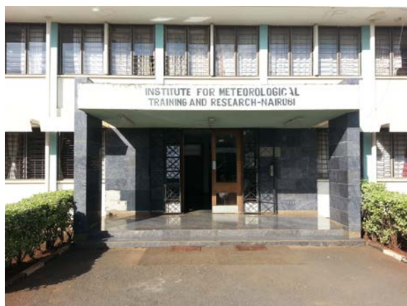
IMTR Administration Block
