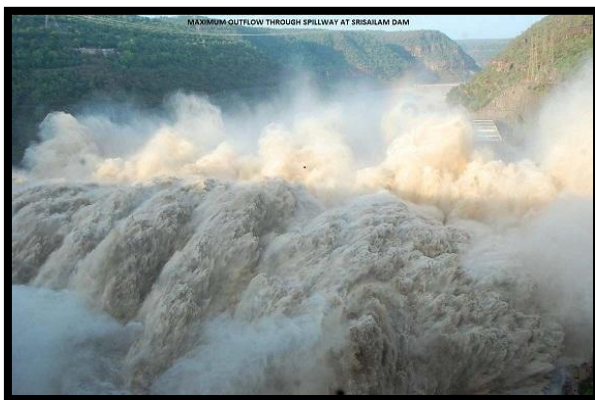
Fig.10 Maximum outflow through spillway at Srisailem dam
