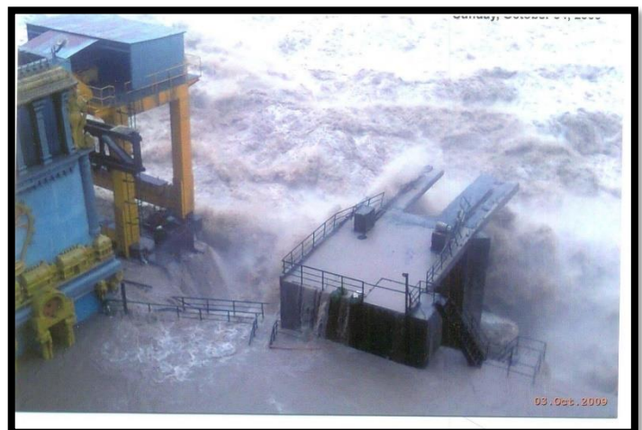
Fig.5 Inundated Power house at Srisailam dam
