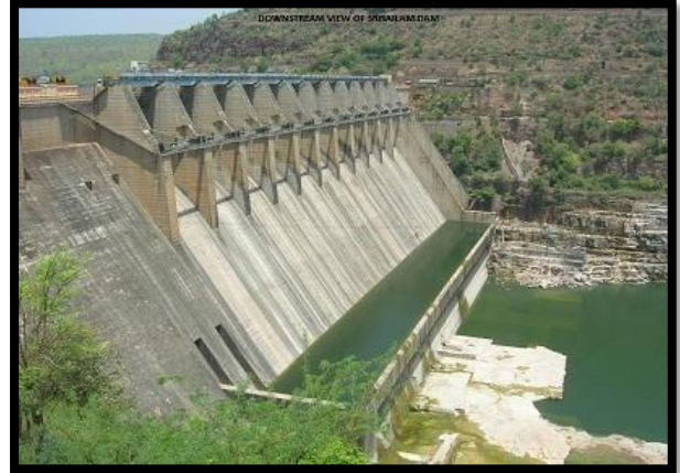
Fig.7 Downstream view of Srisailem dam
