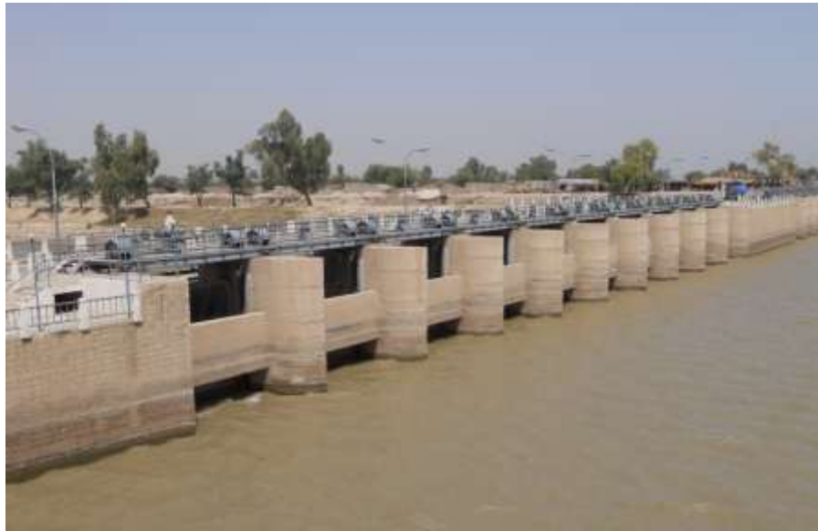
Fig 1: Typical Barrage cum Bridge.
