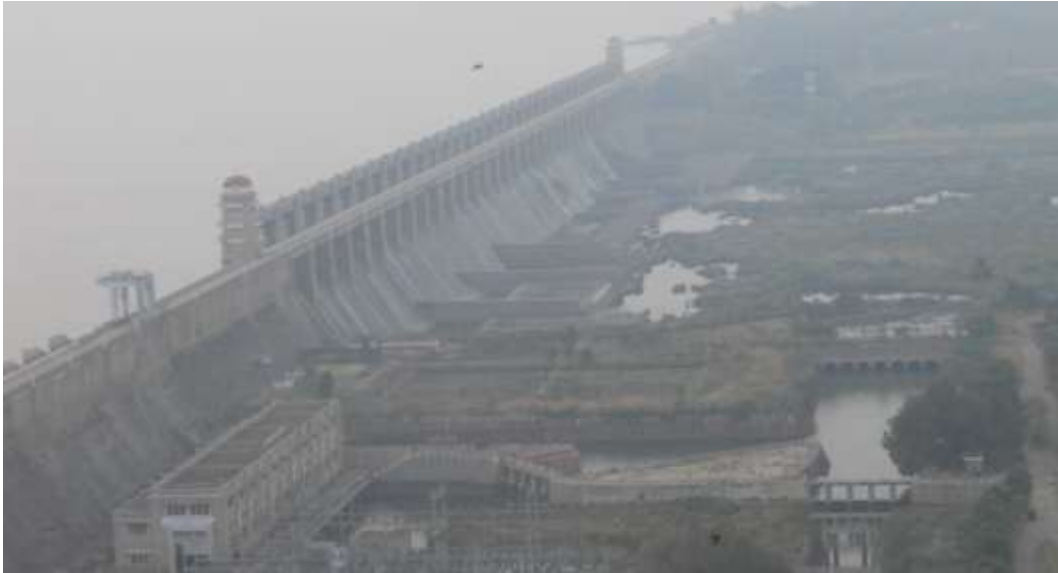
Fig (c) Gravity Dam
