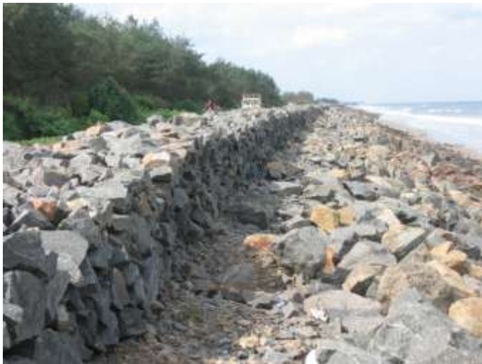
ROCK PACKING NEAR SEA COAST TO PROTECT EROSION IN UPPADA
